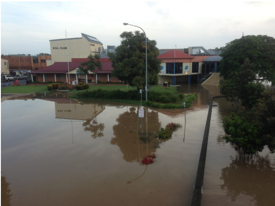
Kempsey levee, Macleay River, 7.55 am, 23 February 2013
