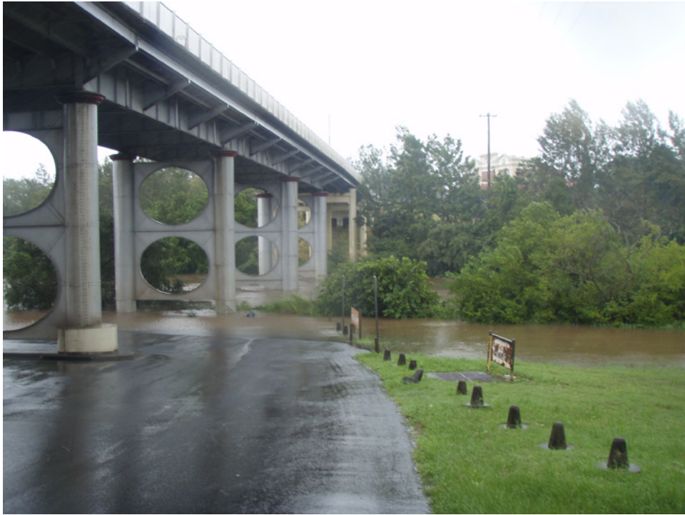
Lismore Bridge, Wilsons River, 8.40 am, 27 January 2013
